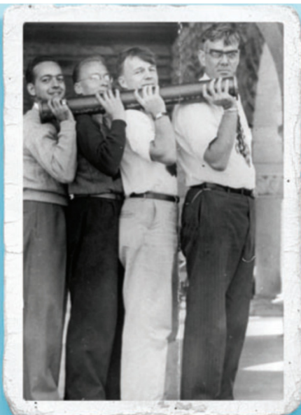
Mark I accelerator section: Professor William W. Hansen (right) of the Stanford Physics Department and three of his graduate students: (left to right) Stanley Kasei, Clarence Carlson, and William Kennedy. They are holding one of the first sections of the first Stanford traveling wave electron linear accelerator. Eventually 3.6 m long, the Stanford Mark I could accelerate electrons to an energy of 6 MeV. The Mark I was followed in 1949 by the Mark II, which was a prototype of one of the sections of a planned, much larger machine, the Mark III. Built under the direction of R. F. Post, the Mark II was first successfully operated in October 1949. Source: SLAC Archives, ARC127, Slide 2; Stanford photo
