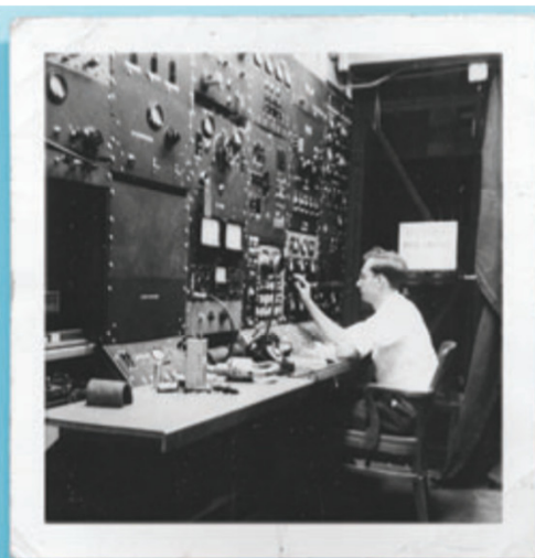
Mark II accelerator control room: Karl Brown at the klystron controls for the Mark II accelerator at Stanford University. Source: SLAC Archives, ARC490; Vera Lüth photo
